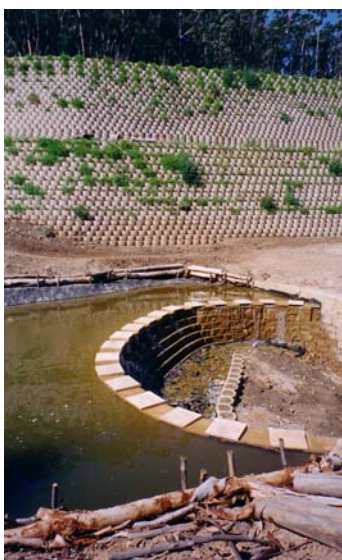
Weir and 12m high retaining wall
