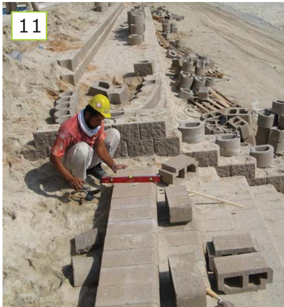
Image 11: Terrace walls complete in the background and stairs almost at final level.
