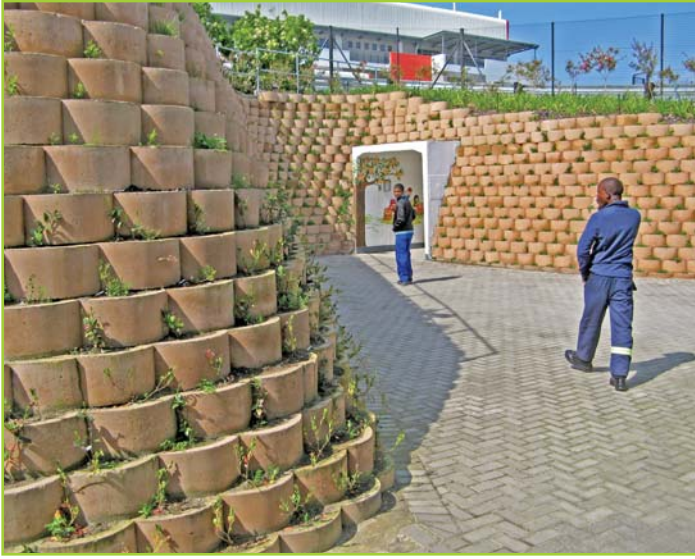
CURVED ROUND FACE WALL, SHOPRITE STORAGE FACILITY
