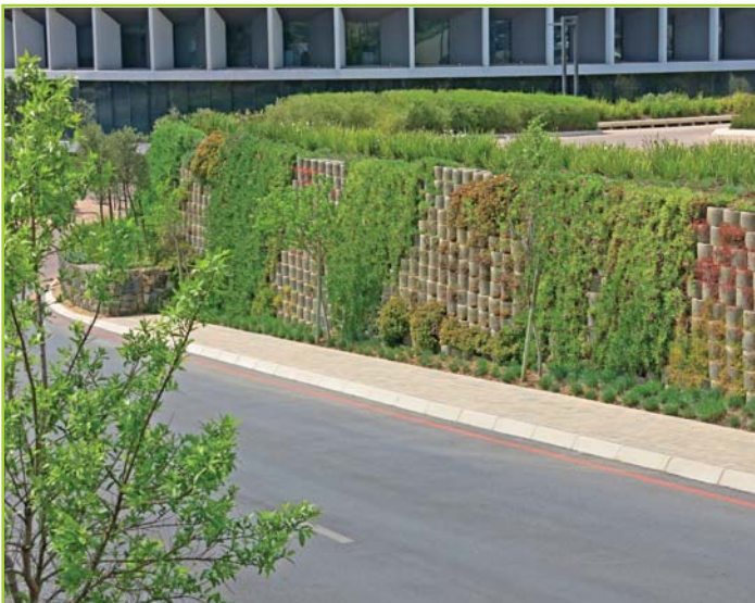
PLANTED SLOPE STABILISATION, CELL C HEAD OFFICE
