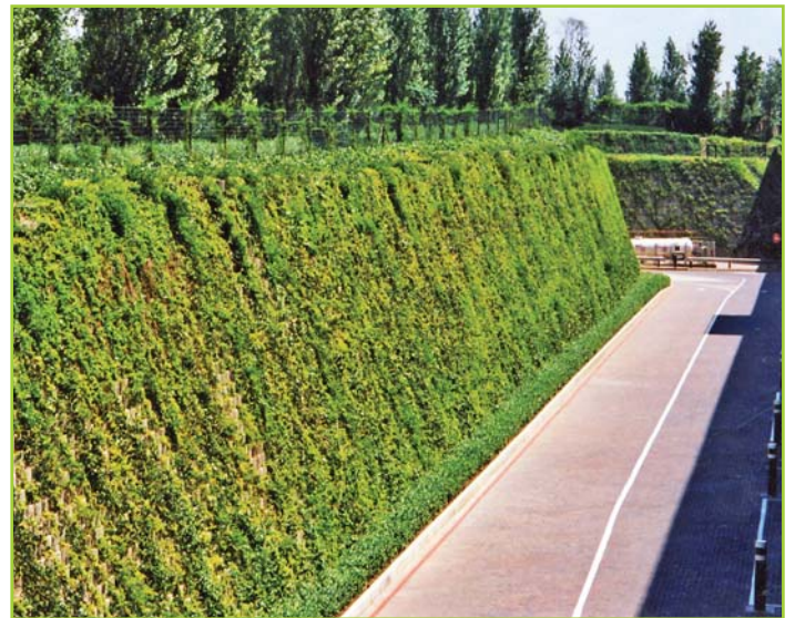
COMPOSITE, PLANT SUPPORTIVE ROADSIDE WALL
