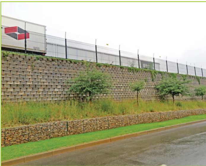
WAREHOUSE RETAINING WALL, WITH GABIONS
