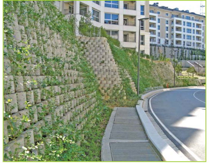
PLANTED SLOPE EROSION CONTROL, OFFICE BLOCK
