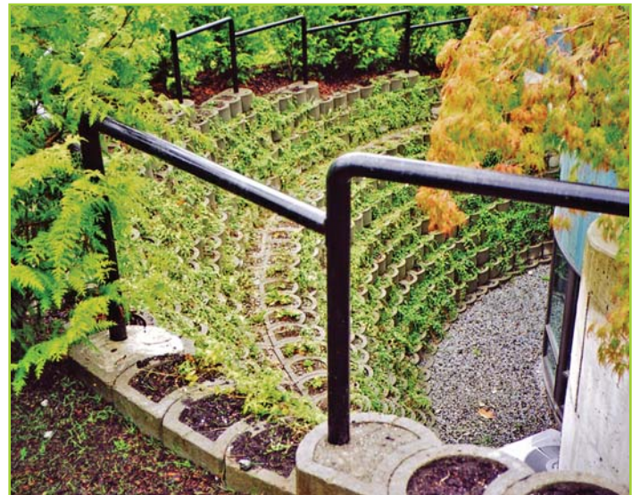
CURVED RETAINING WALL AND RAILINGS
