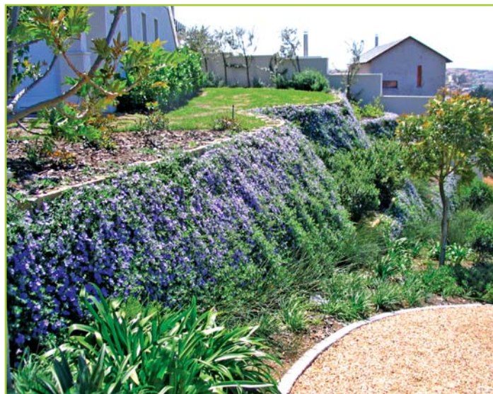
A TERRAFORCE WALL WITH PLANT COVER IN FULL BLOOM
