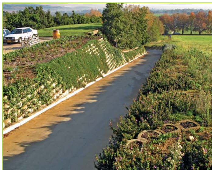
ROUND FACE ROADSIDE RETAINING WALLS, WINE ESTATE
