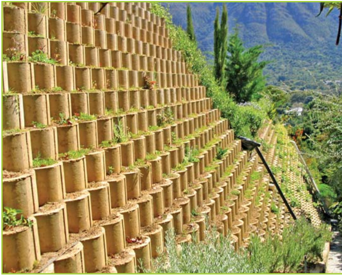
HIGH COMPOSITE RETAINING WALL
