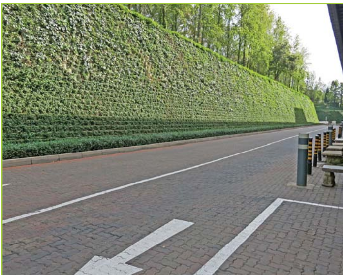
ROADSIDE RETAINING WALL WITH FULL PLANT COVER
