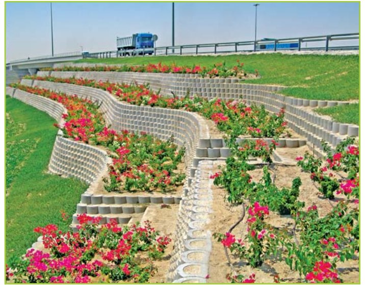
CLOVER LEAF INTERCHANGE RETAINING WALL, QATAR
