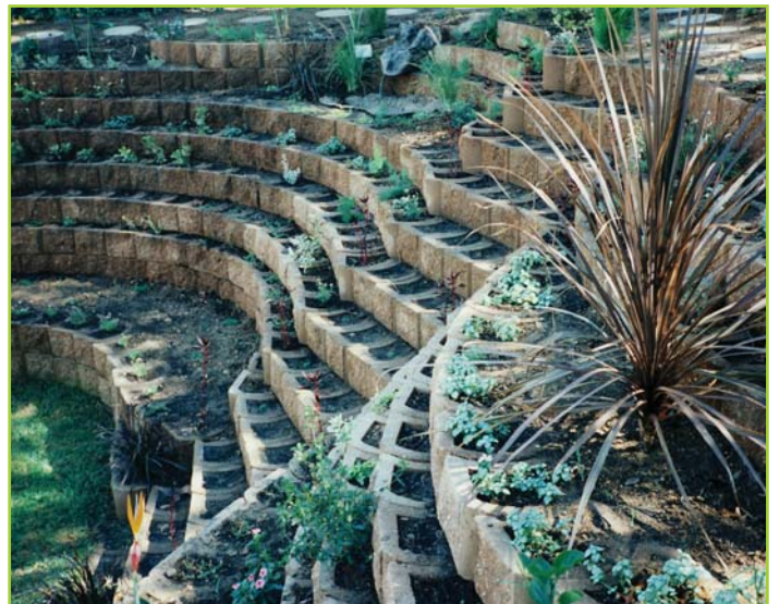
PLANT SUPPORTIVE SLOPE PROTECTION
