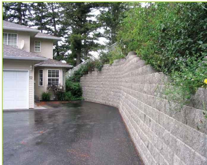
NEAR VERTICAL, COMPOSITE WALL
