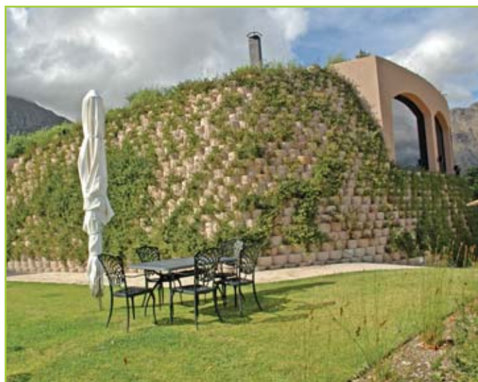
ROUND FACE WALL FOR RESTAURANT SET INTO FILL SLOPE
