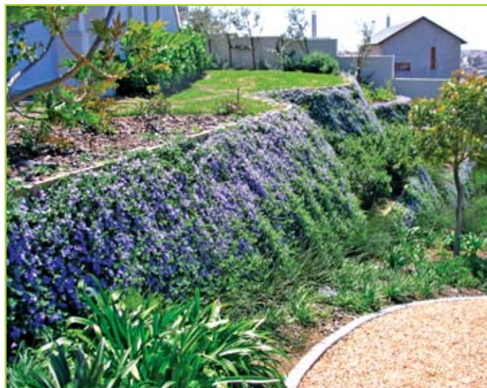
A TERRAFORCE WALL WITH PLANT COVER IN FULL BLOOM
