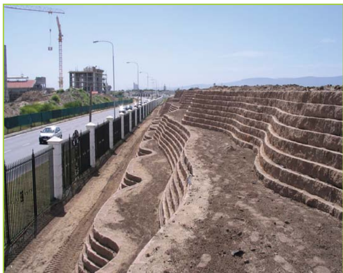
MEANDERING TERRACES FOR NOISE BARRIER
