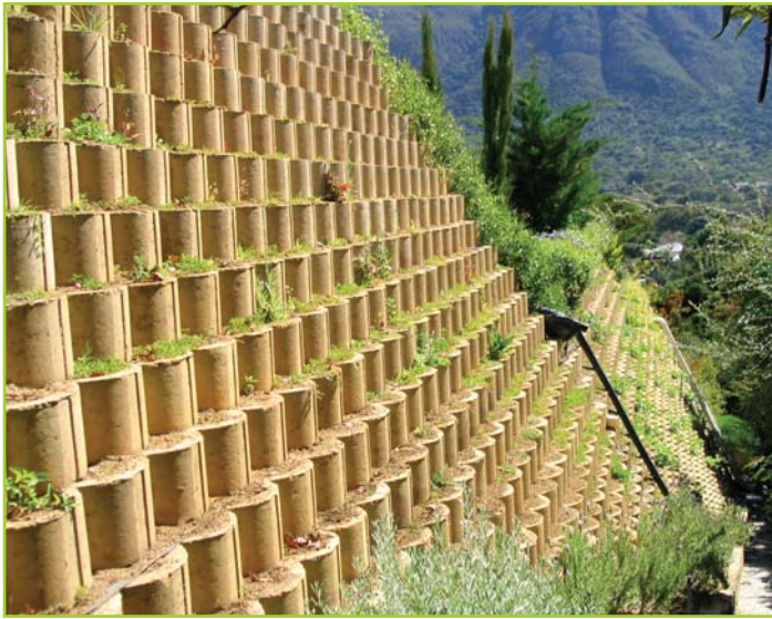
HIGH COMPOSITE RETAINING WALL
