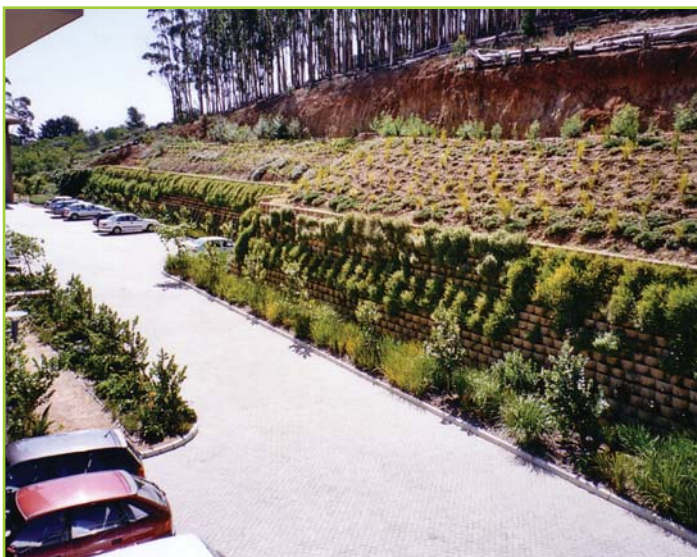
COMPOSITE RETAINING WITH TERRACING AND PLANT COVER
