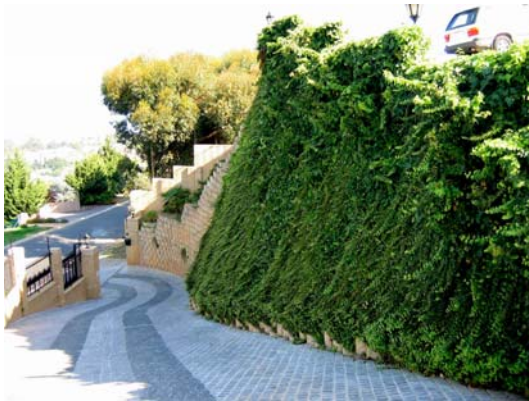
Contractor: Terrafirma cc
