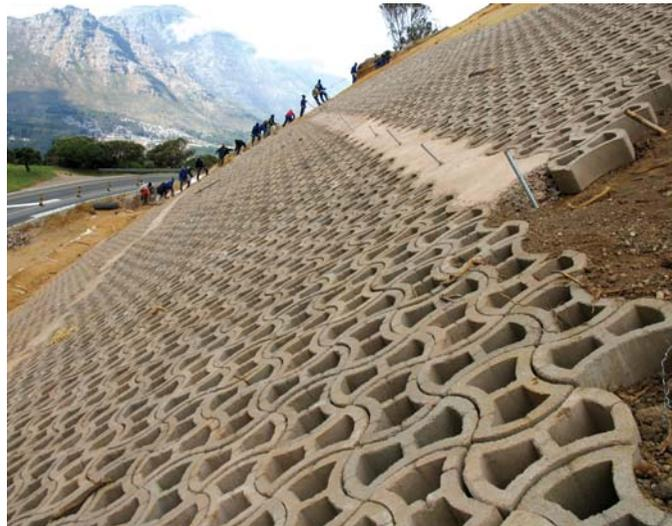
23064 blocks were used to stabilise this slope
