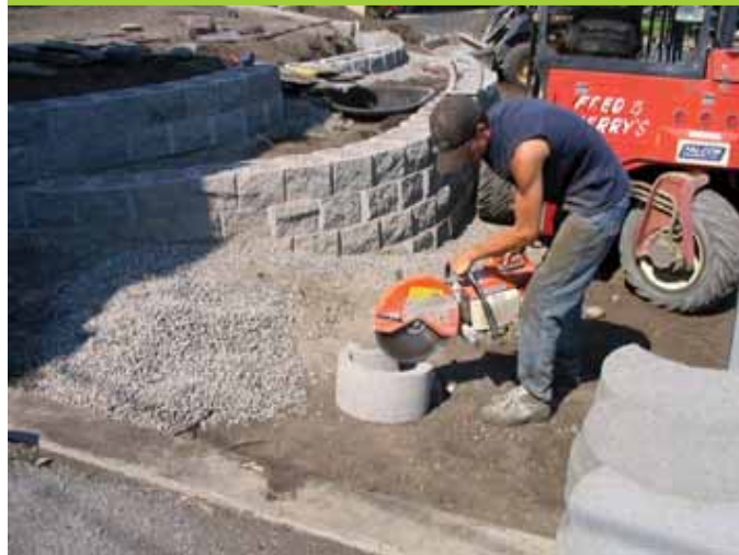
Precision cutting of blocks to shape
