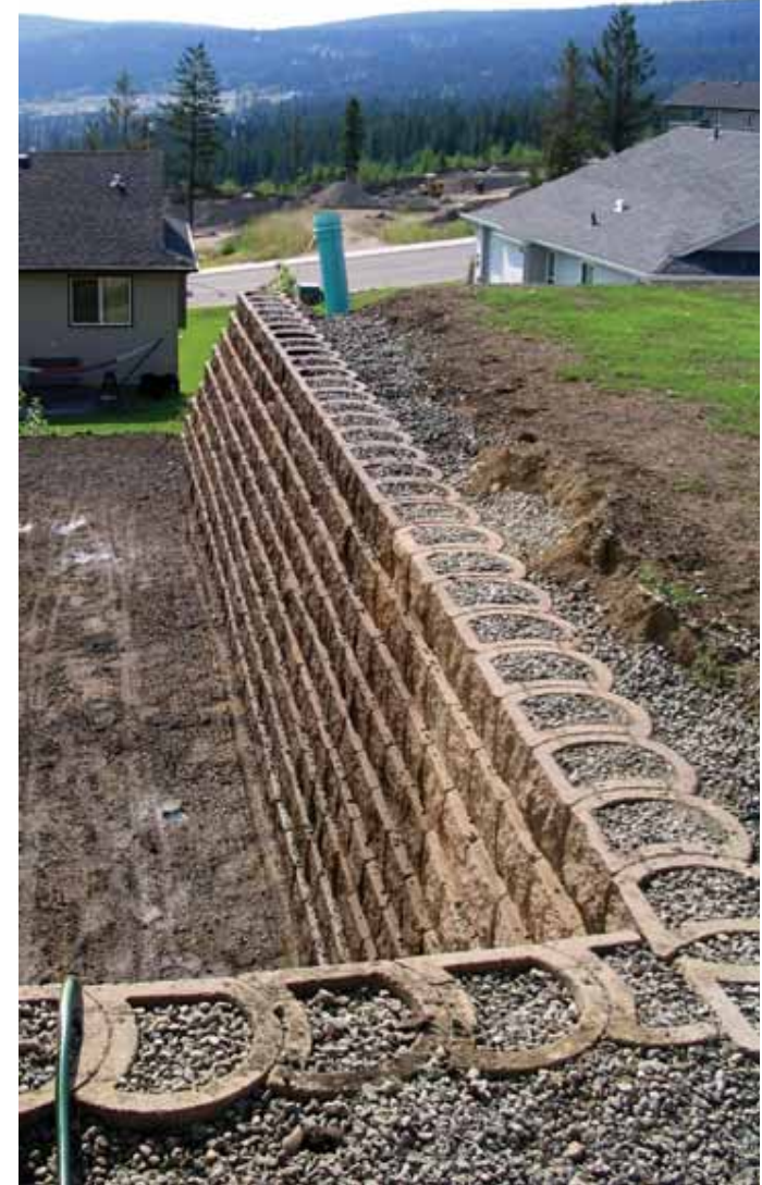
Steep, low maintenance wall with neat corner detail
