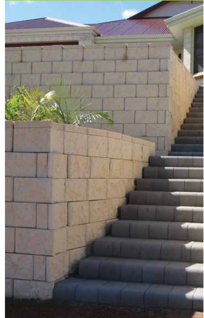
Neatly cut corners, stabilised with cement/sand backfill.
