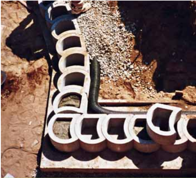
Corner blocks filled with concrete and drainage installed.
