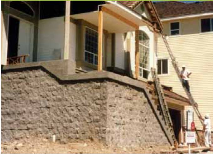
Architectural features are easily achieved with concrete filled blocks.
