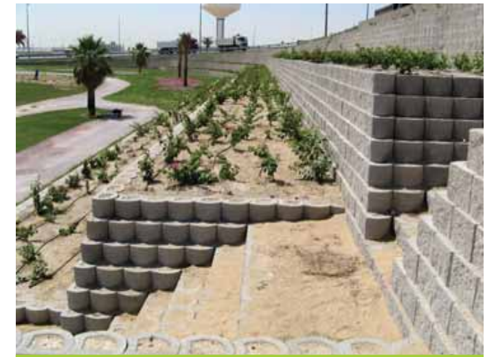
Bryan's maintenance step innovation
