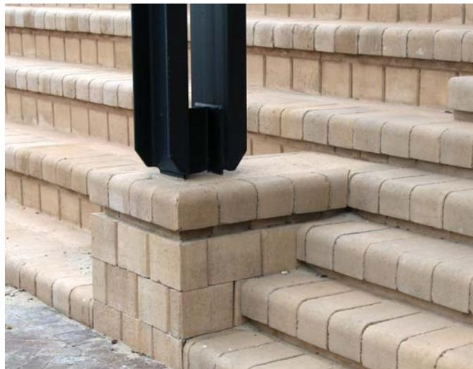
4x4 blocks cut to shape and size to create the column foundation
