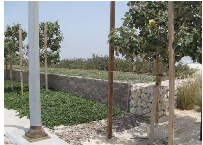
Vertical Terraforce toe walls with gabion protective cross barriers. Plants established
