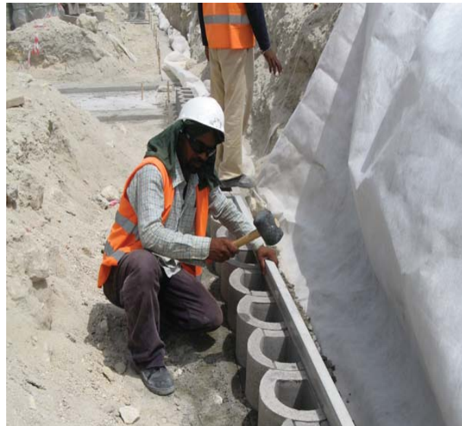
First course placed to line and level. Geofabric backing in place.
