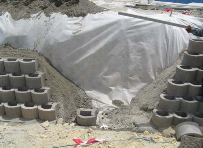
Lines installed longitudinally with gaps at specified centres for access stairs.
