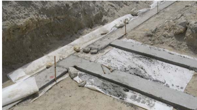
Concrete levelling pad on geofabric on compacted gravel
