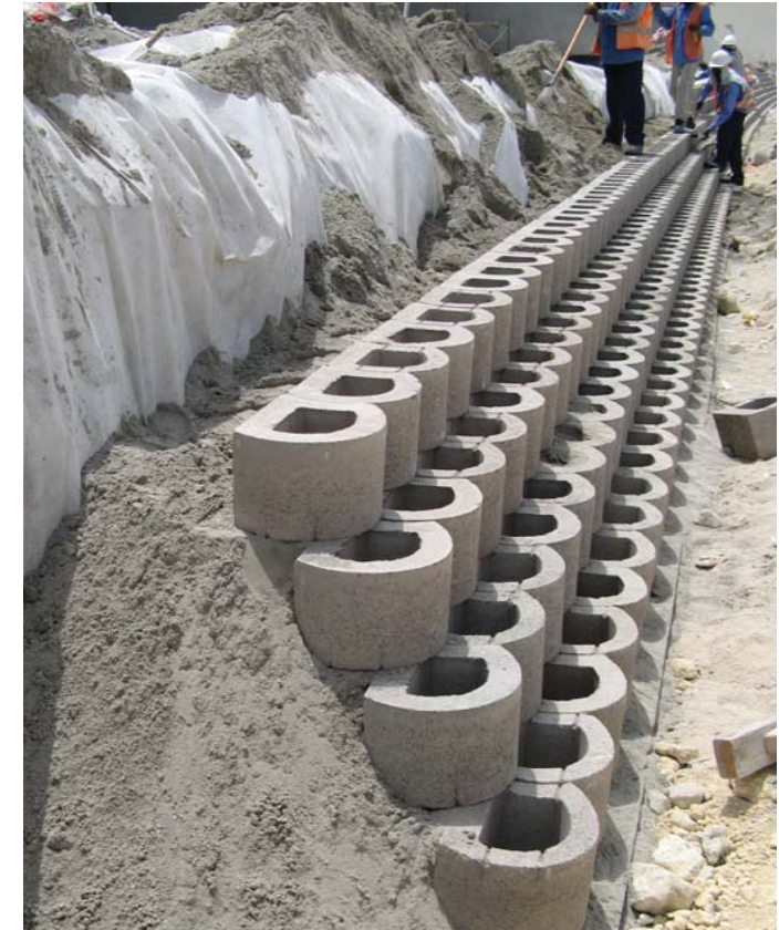
Line 4 installed with backfill as specified and compacted, Round-face option.
