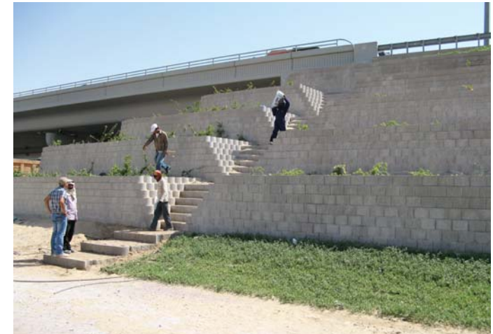
Maintenance in progress
