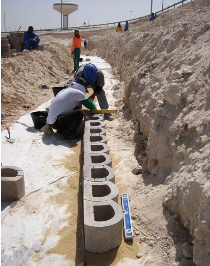
First blocks laid onto goetextile foundations
