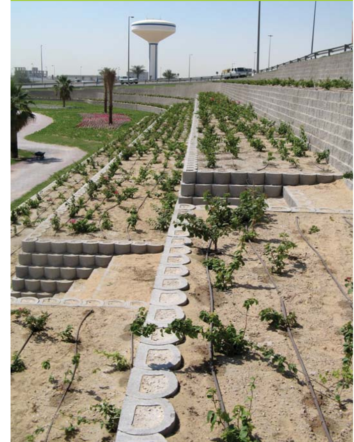
Completed wall with plants, irrigation and stairs
