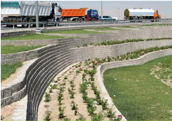
Interchange with rock-face elevation
