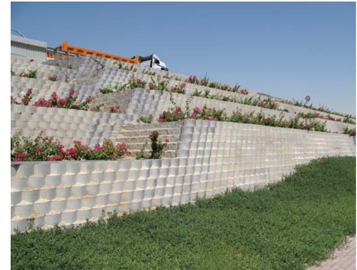
Stepping up of terraces to match ground profiles
