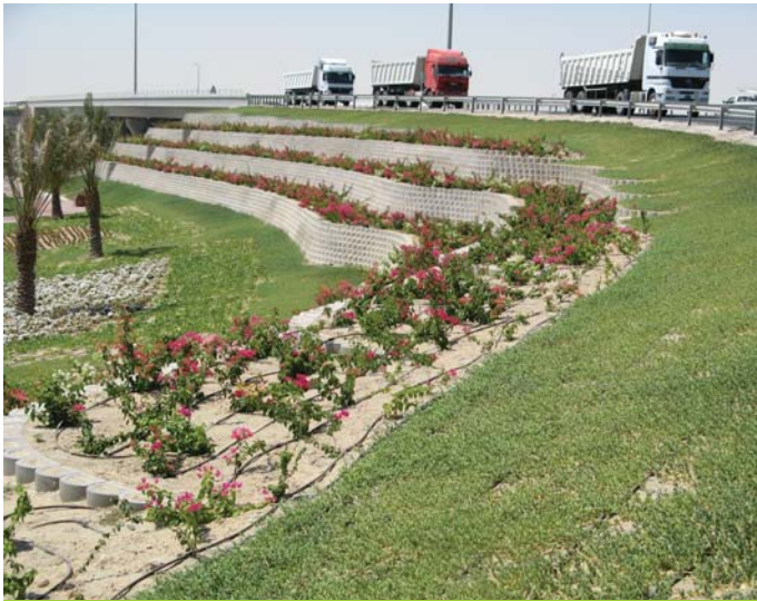
Completed wall with plant cover
