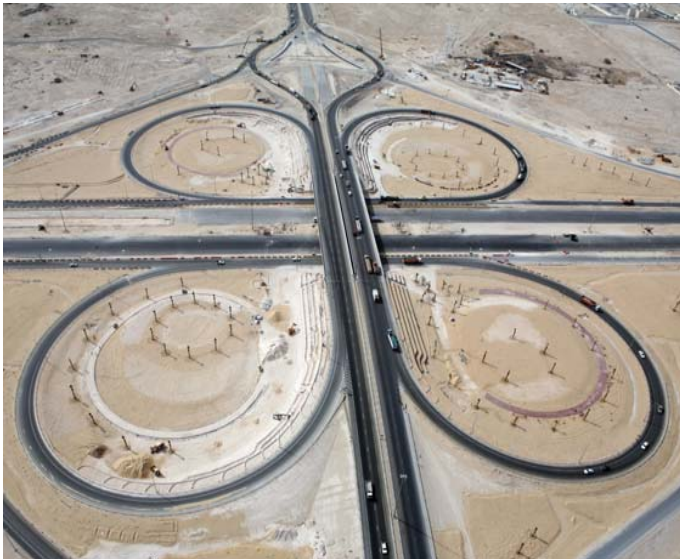
An aerial view of interchange 24. The terracing on each loop is already visible.
