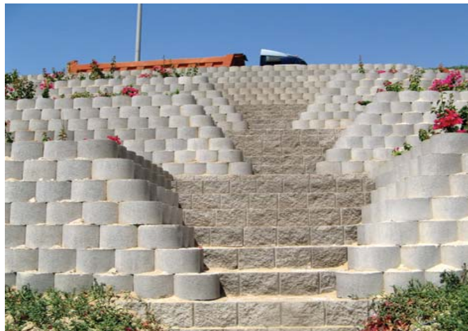
Detail of maintenance stairs
