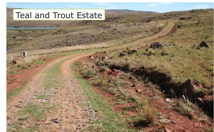
of road stabilization to be indispensable in wet rainy weather. It completely halts erosion and also looks very neat. Much more pleasing than soil or gravel roads, which are so prone to soil erosion. Traction for vehicles is enhanced considerably as well."
