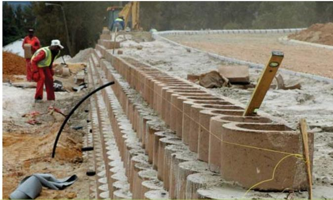
To check row levels, a string is run along the top of the row under construction.
