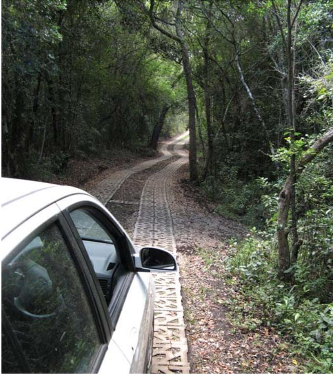
soil. In general though, repair and maintenance of the road is kept relatively simple. When subjected to heavy loads, the occasional block may crack and can then be left in place for a while to still function perfectly or it can be replaced with a new block.
