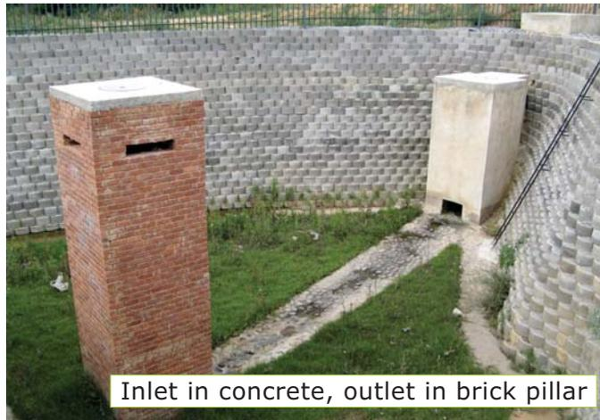
Inlet in concrete, outlet in brick pillar
