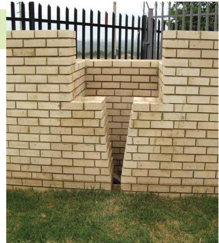
V-shaped outlet and trash trap behind A 25 mm storm filled the pond 2 bricks high.
