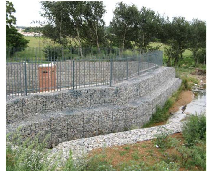
Attenuation pond, with gabions and Terraforce L11 blocks next to a small stream, which as a result gets protected from stormwater damage.
