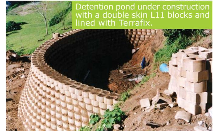
Detention pond under construction with a double skin L11 blocks and lined with Terrafix.
