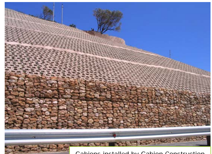
Gabions installed by Gabion Construction
