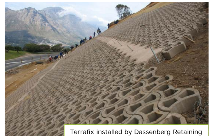
Terrafix installed by Dassenberg Retaining
