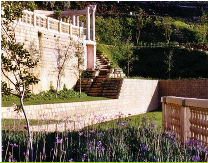
6m high vertical, composite wall
