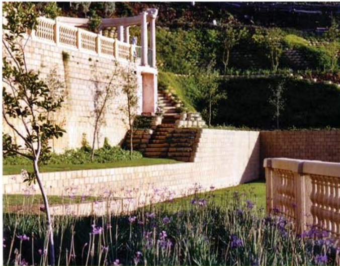
6m high vertical, composite wall
