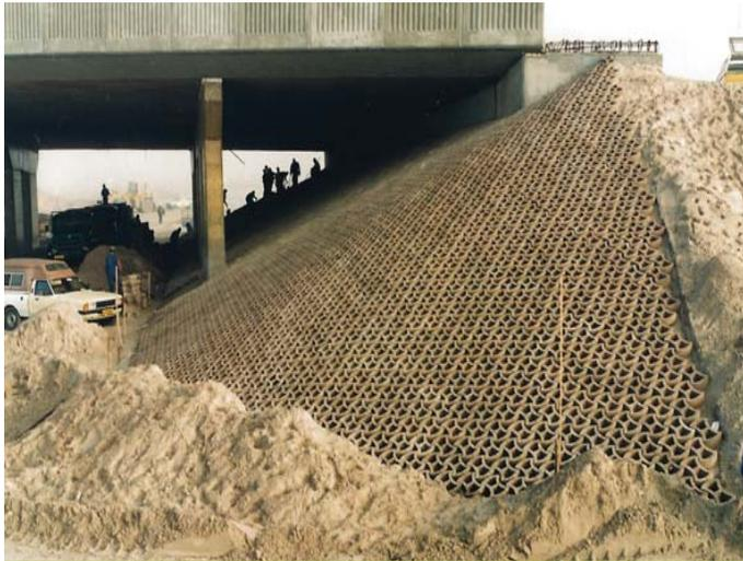
**Sandy bridge abutment retained with a permeable surface**
