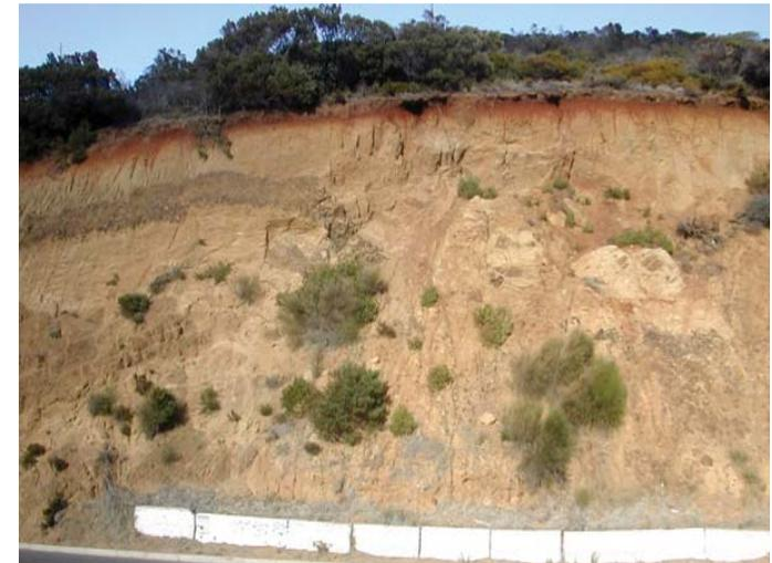
Heavily eroded cut slope posing a danger to passing traffic
