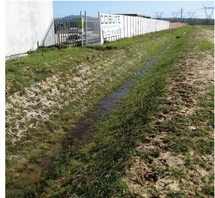
**Permeable erosion control of a storm water channel with grass cover**
