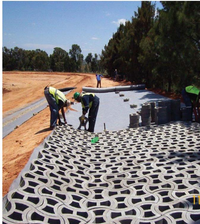
**Permeable erosion control at a waste site**
