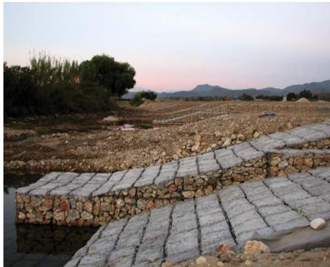
Gabion groynes with concrete panels to protect against abrasion
