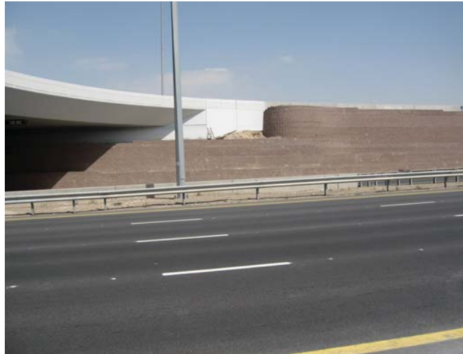
Mirdif Interchange Dubai. Terraforce L16, Consent LLC
