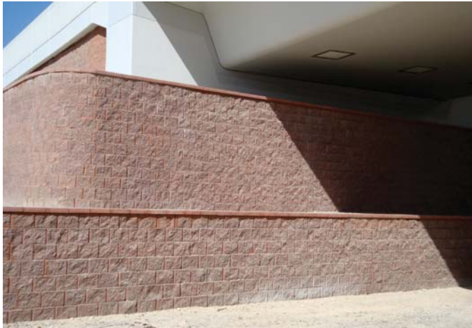
Terraforce L16 retaining walls with capping stones
