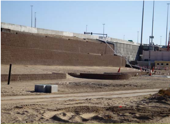
Mirdif Interchange, near vertical Terraforce terraces, 9300m 2
