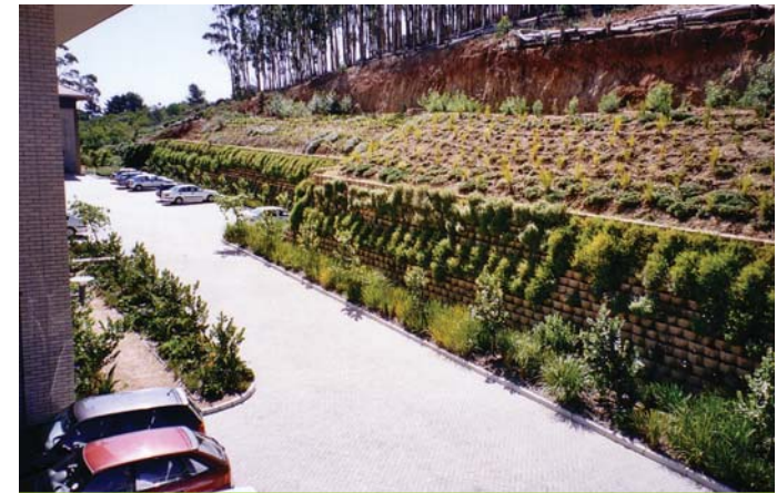
Retaining for 5m high x 95m long embankment
