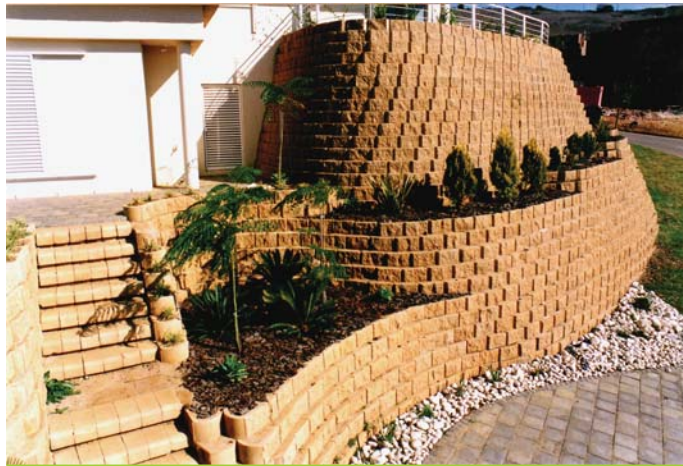
6m high split face L11 block wall
