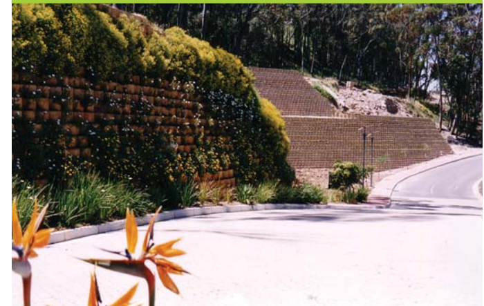
Retaining for 5m high x 95m long embankment
