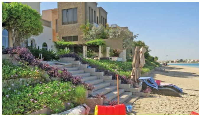
Good plant cover on one of the walls
