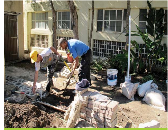
Digging out the 100mm foundation
