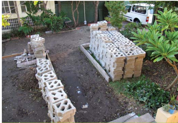
Stack blocks neatly on an even surface
