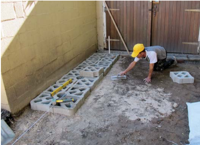
Levelling the sand bedding layer
