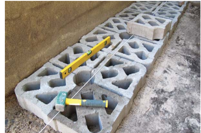
Packing the blocks to line and level
