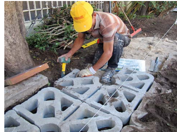
Joe tapping the blocks into position
