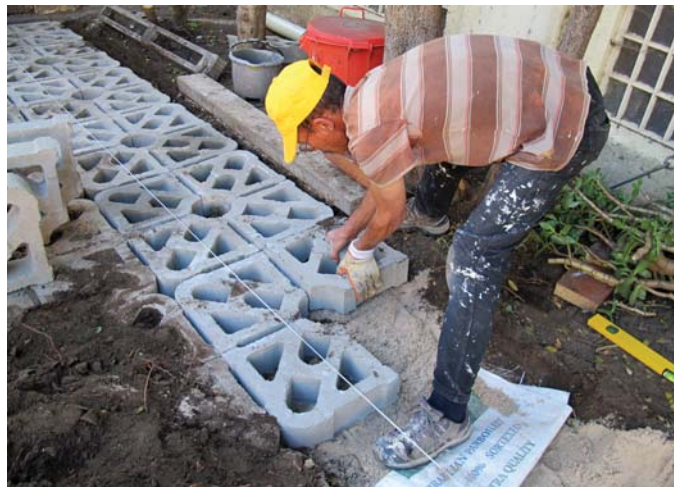
Packing the blocks with a small fall towards the drainage channel
