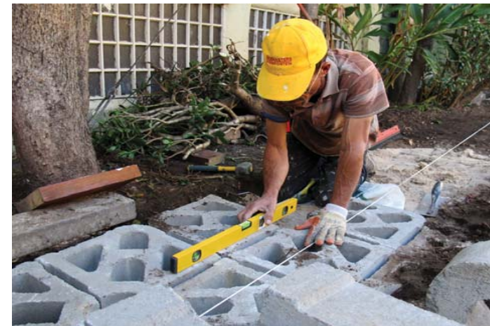
Checking the fall with a level
