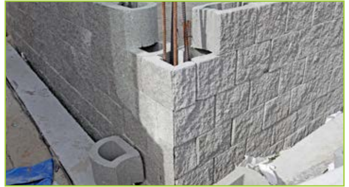
REBAR REINFORCED CORNER
