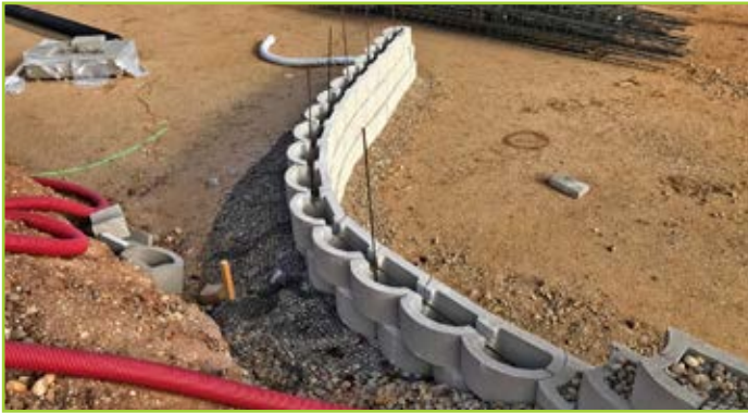
HORIZONTAL AND VERTICAL REBAR
