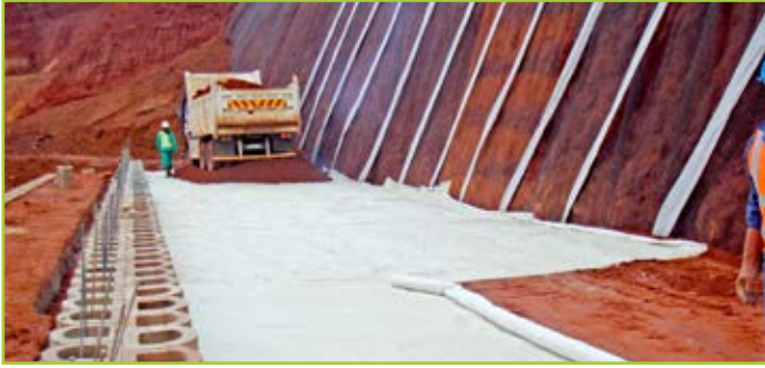
RC FILLED WITH GEOFABRIC
