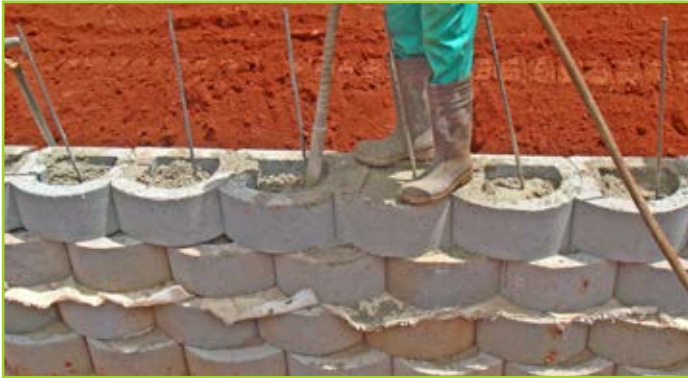
COMPACTING CONCRETE INFILL IN BLOCKS
