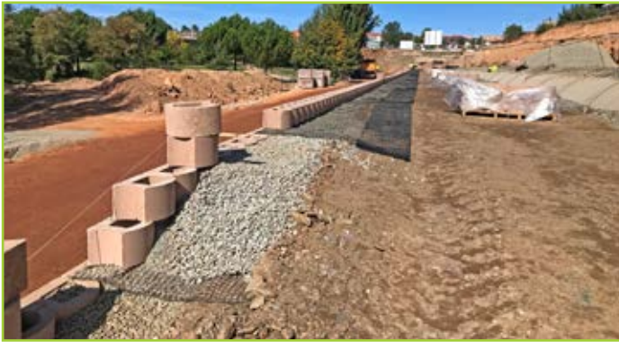
GRAVEL FILLED WITH GEOGRID
