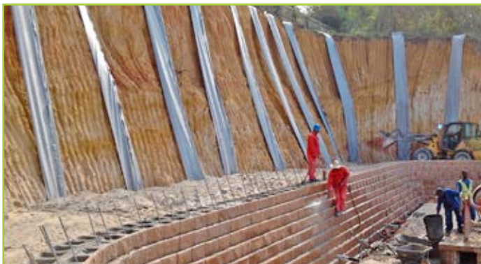
EXTRA HEAVY DUTY EARTH RETAINING
