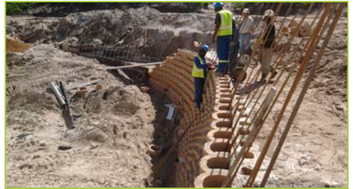
SLOPING RC FILLED WALL
