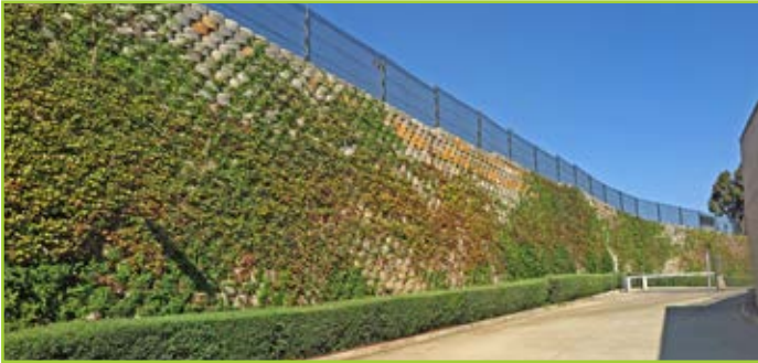
STEEP ROUND FACE WALLS, FULLY PLANTED
