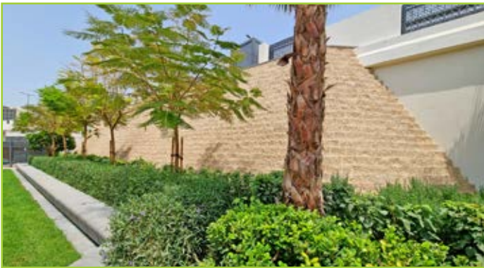
BRIDGE ABUTMENT ROCK FACE WALLS DUBAI
