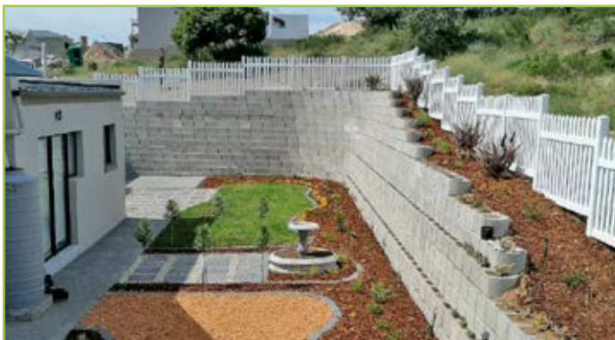
FLAT FACE WALLS, PRIVATE RESIDENCE
