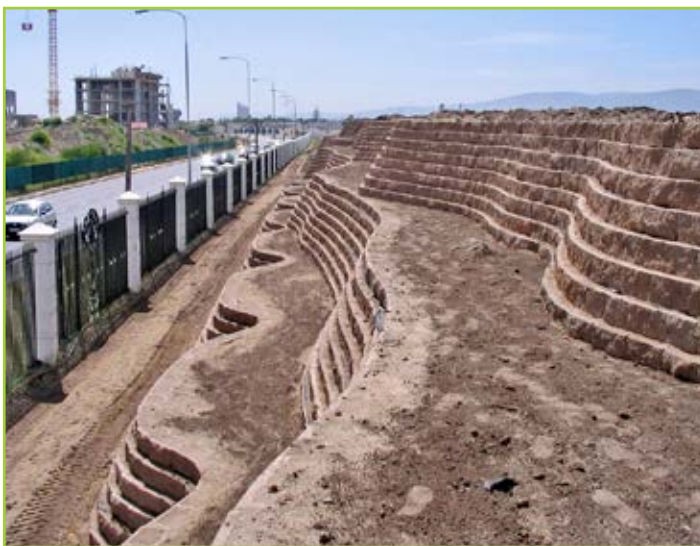
Noise barrier before planting and irrigation at the Oasis Retirement Village, South Africa
