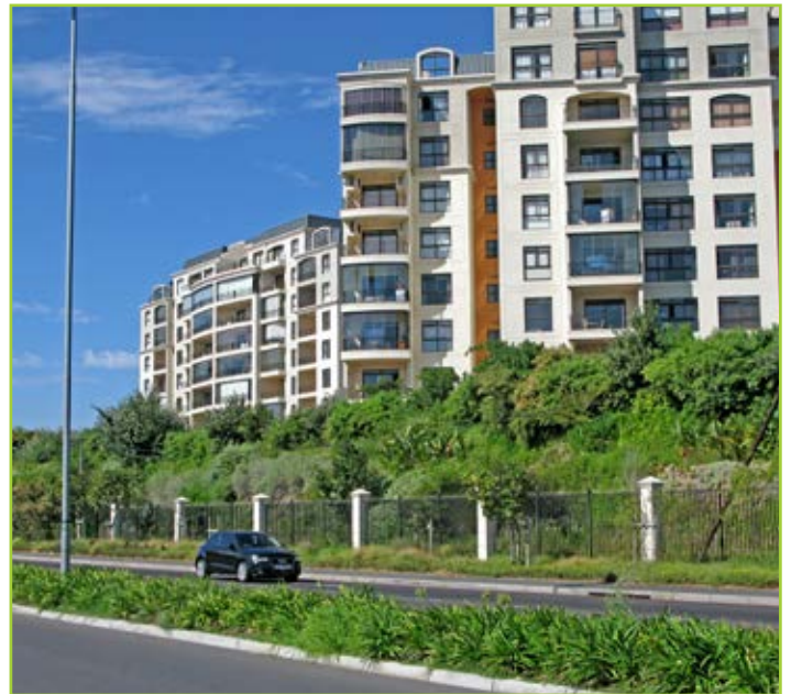
The planted wall offers traffic noise mitigation adds an extra layer of security
