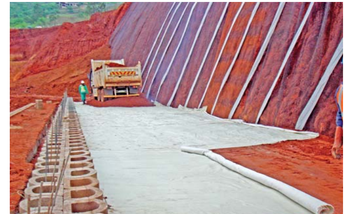
Geogrid clamped between the blocks
