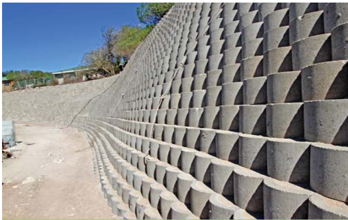
Single skin wall, cement stabilised back-fill
