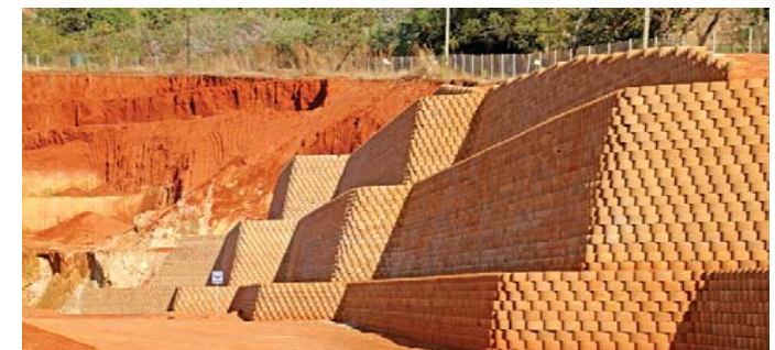
The wall 50% completed
