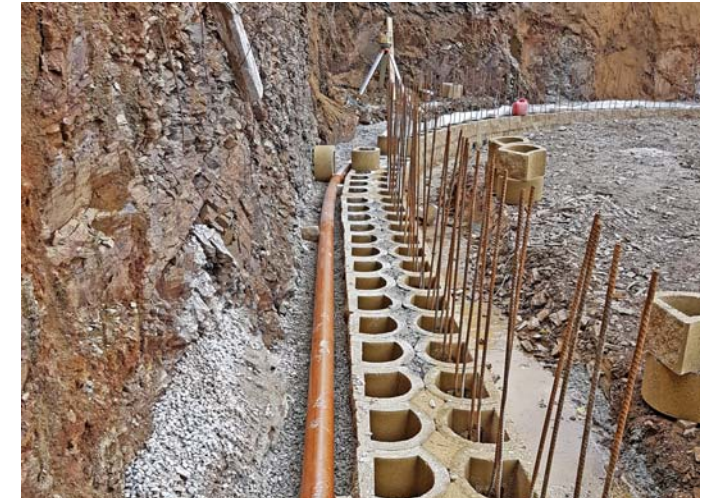
Foundation with protruding re-bars
