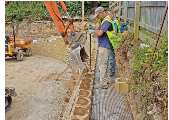
Geogrid reinforcing is placed at intervals
