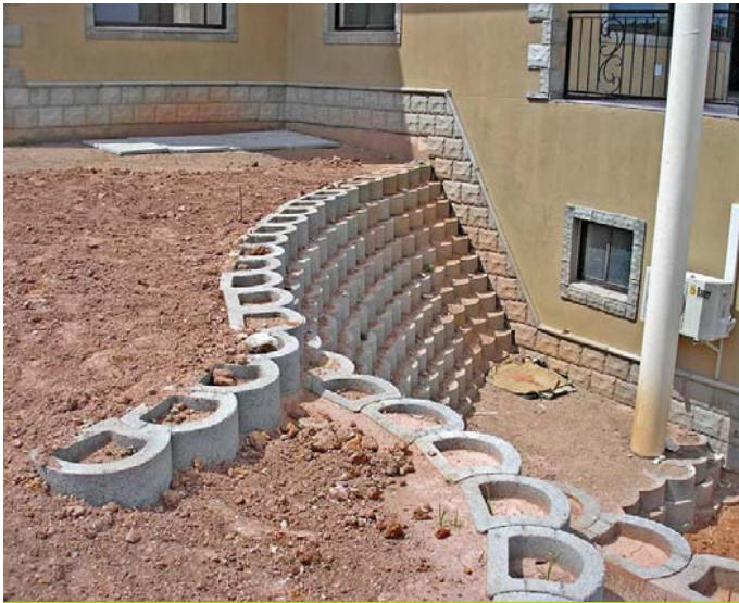
Gravity retaining Terraforce wall
