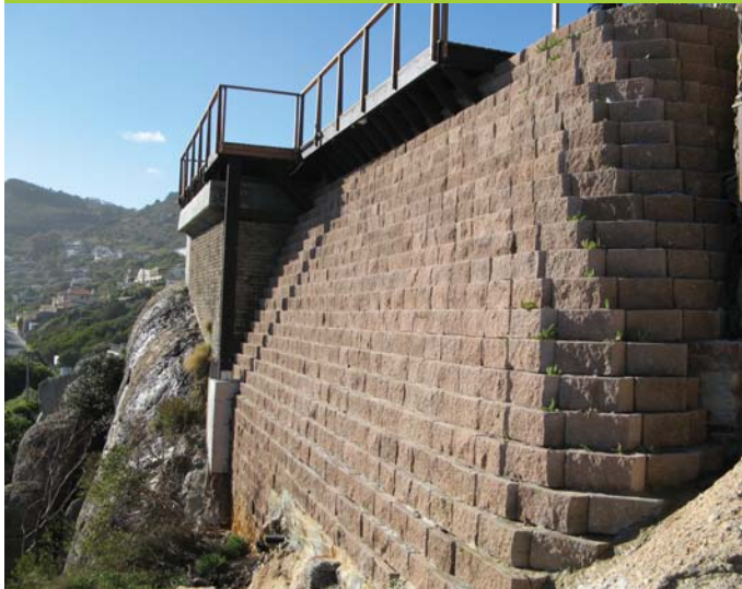
The Retaining wall under the pool
