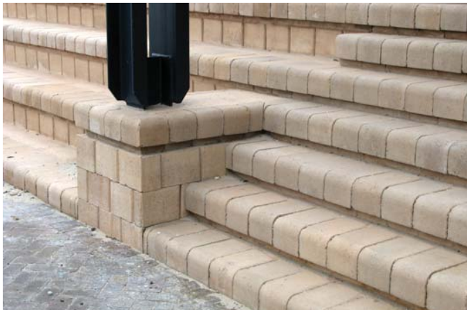
Intricate detailing by Dassenberg site agent Georg Brand.
