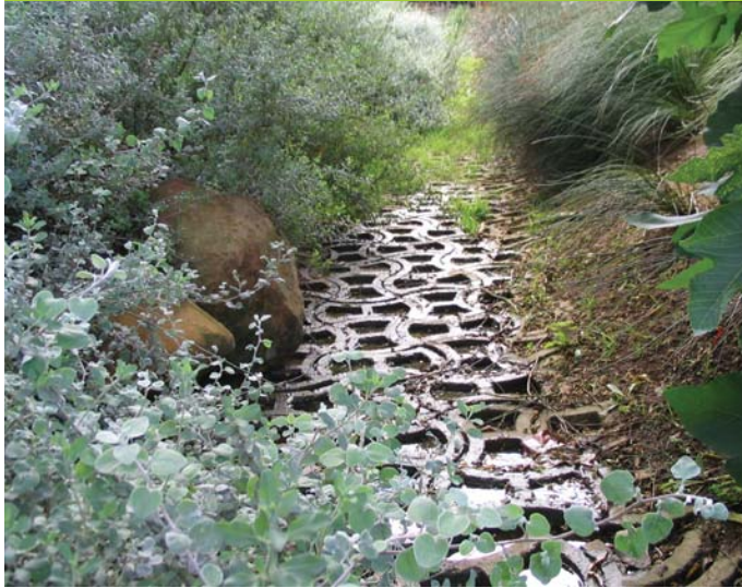
The stream lined with Terrafix blocks
