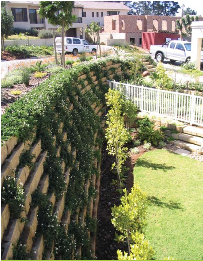
For a steep rock face wall with limited space, trailing plants are suitable.
