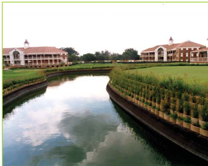
STORM WATER COLLECTION PONDS
