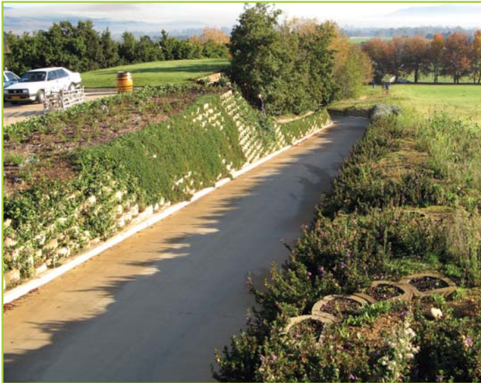
ROADSIDE STABILISATION ON CAPE WINE ESTATE
