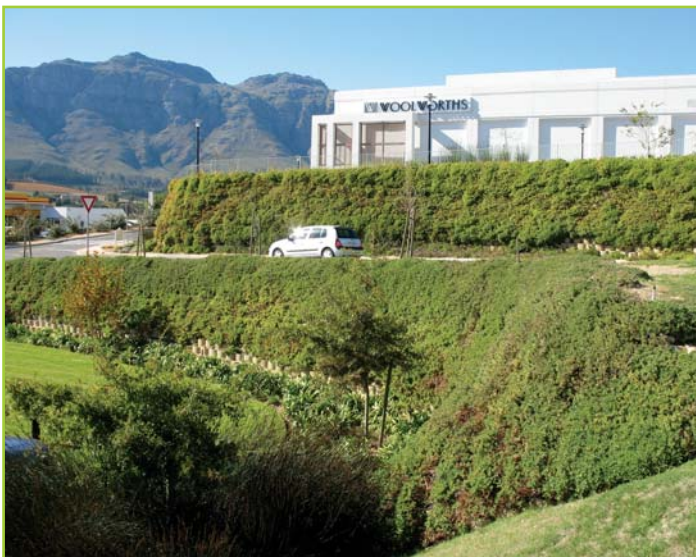
ROADSIDE RETAINING, ROUND FACE BLOCK
