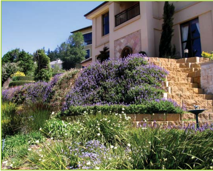
STABILISING AND LANDSCAPING OF CUT & FILL SLOPES
