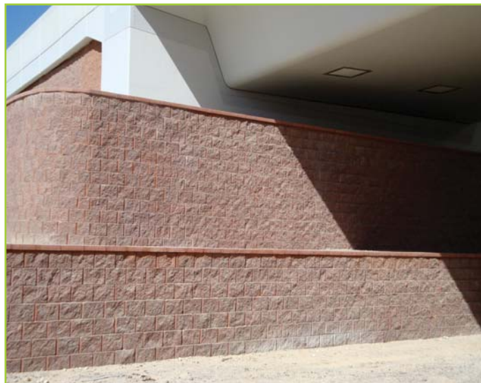
RETAINING WALL AT INTERCHANGE IN DUBAI
