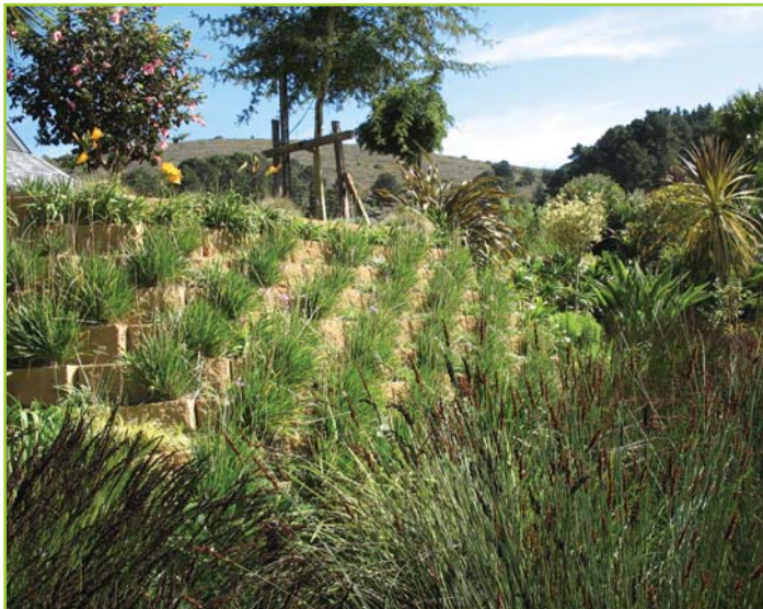
LIGHT GRAVITY RETAINING, PLANT SUPPORTIVE
