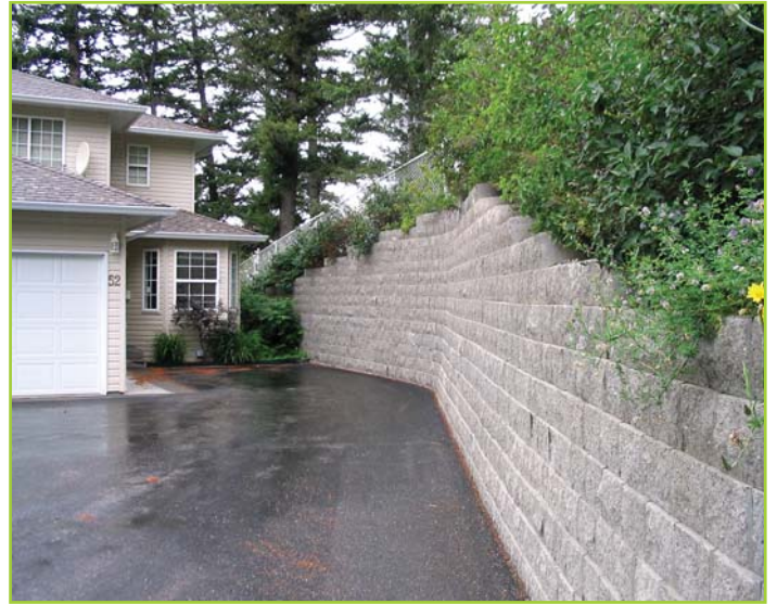
NEAR VERTICAL, COMPOSITE WALL
