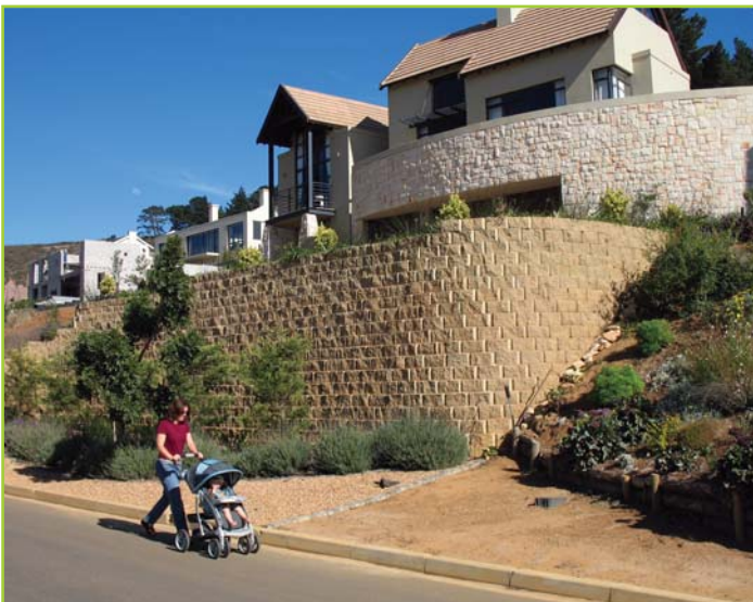
SUPPORTING A NEW DRIVEWAY
