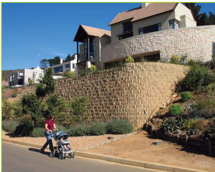
SUPPORTING A NEW DRIVEWAY
