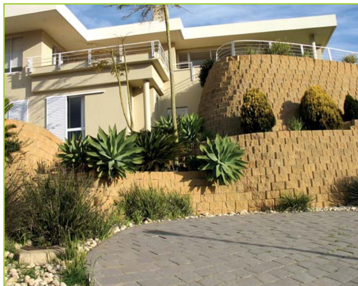
TERRACED COMPOSITE RETAINING WALL WITH FEATURE PLANTS
